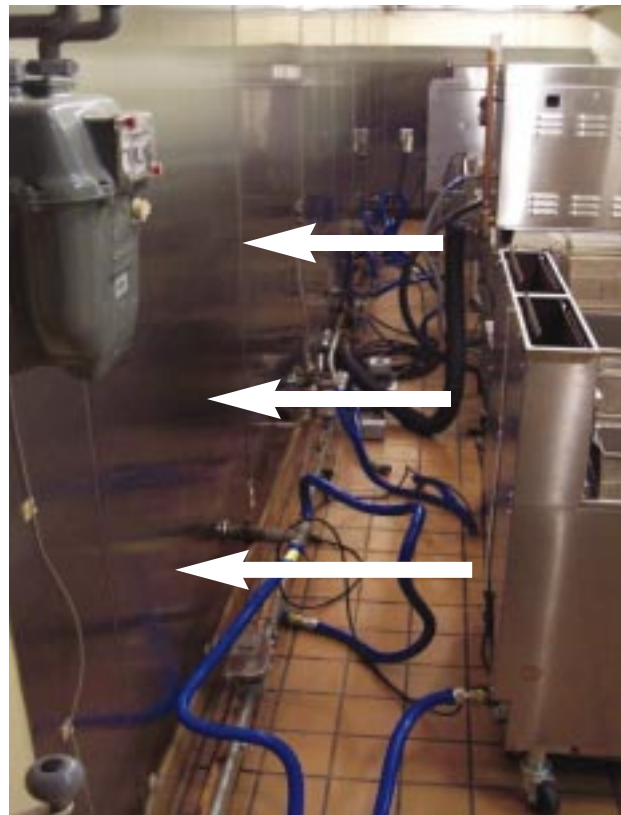
Pushing back the appliances allows for more hood overhang (6 inches is minimum code requirement), which improves capture and containment of cooking effluents and heat.
